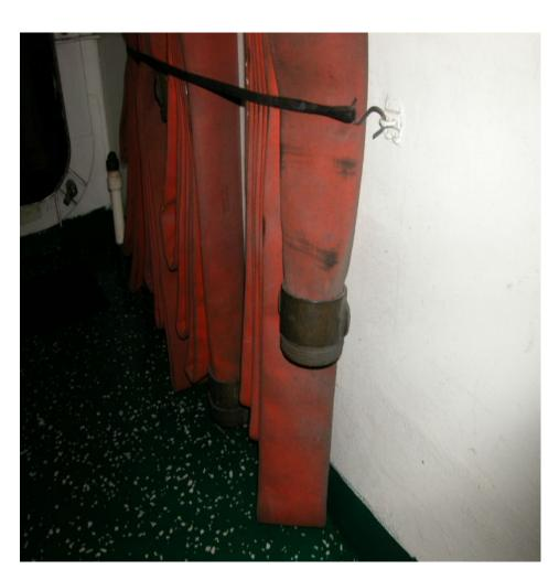
Faked spare hoses need to be stowed with the female on the outside protecting the threads IAW MRC.
