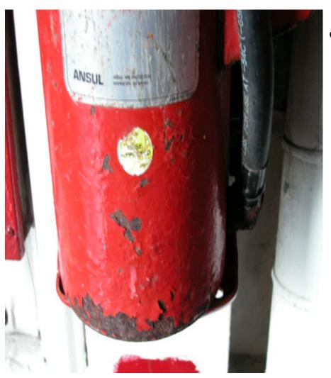
Bottles stowed on or near the weather decks need to be rotated often or covered to avoid corrosion.
