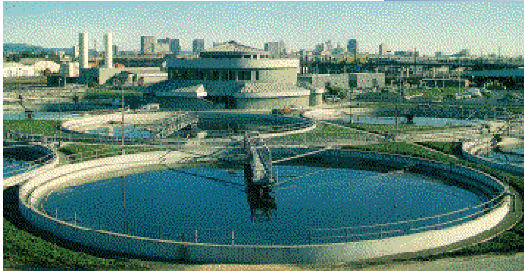
WASTEWATER TREATMENT FACILITY ALAMEDA, CALIFORNIA
