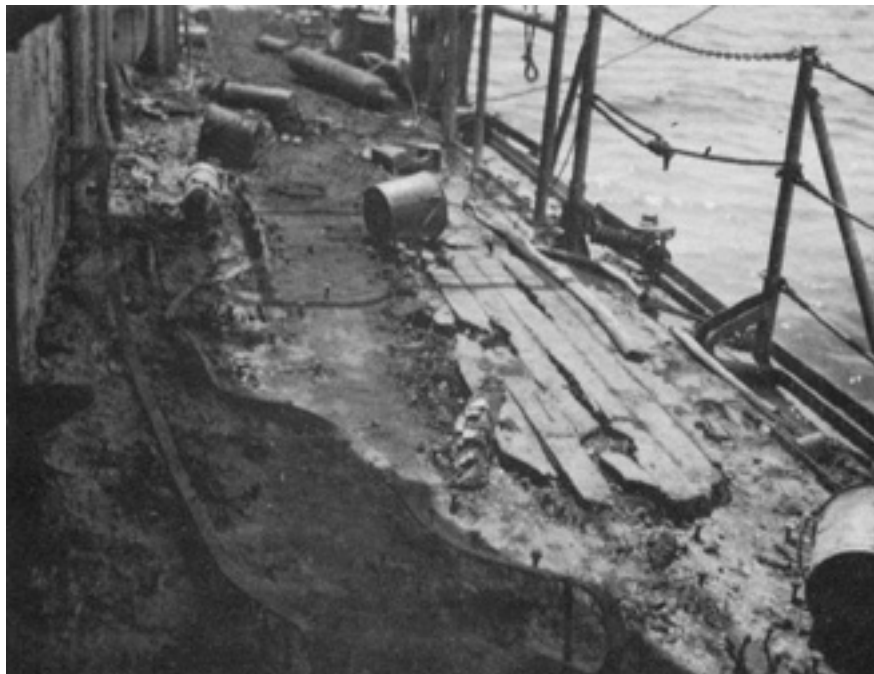
Photo 8: USS ERIE - Main deck abreast after deck house. Note that wood deck has burned.
